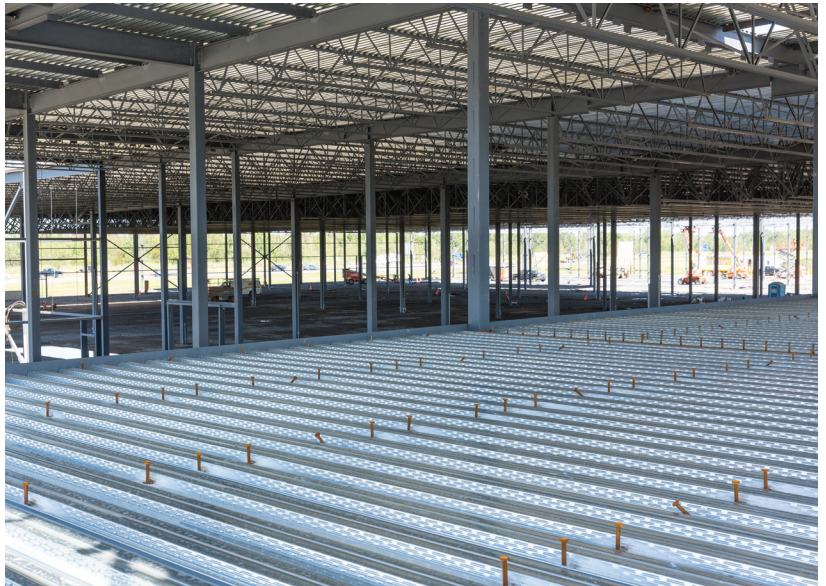
Floor deck ready for concrete placement.
