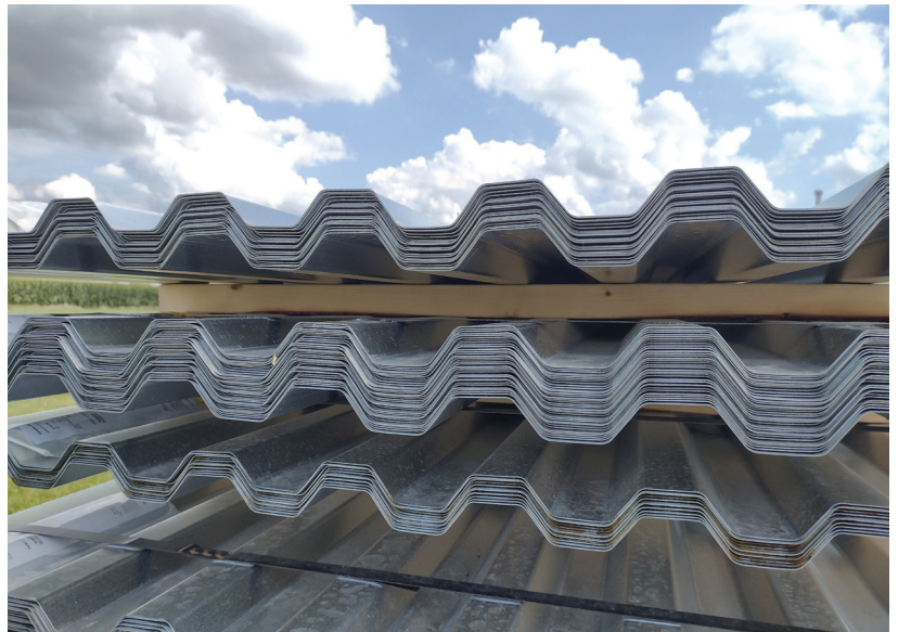
Deck stored on site prior to installation.
