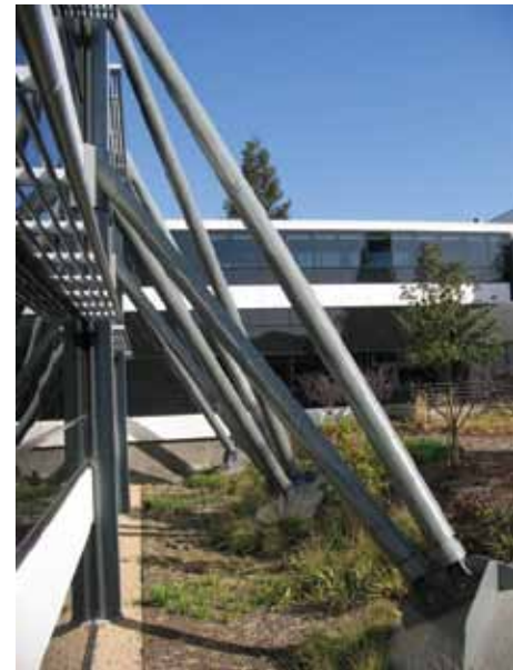
Figure 6: Externally anchored bracing. Courtesy of Mitsui & Co. (U.S.A.), Inc.
