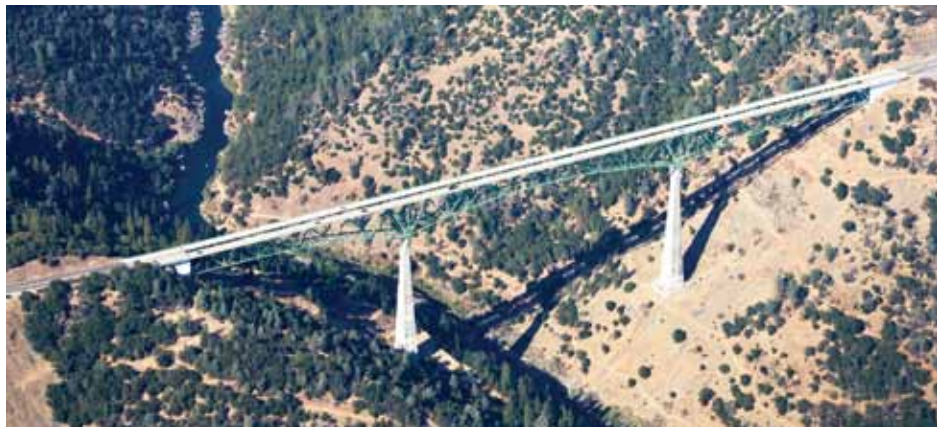
Figure 3: Foresthill Road Bridge. Courtesy of Todd Quam, DigitalSky Imaging.
