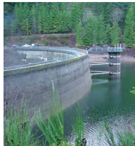
Figure 4: Casad Dam and intake structure. Courtesy of Star Seismic.
