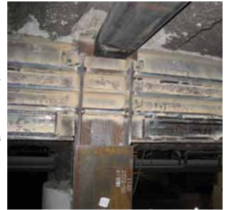
Figure 3: Typical drag retrofit connection.
