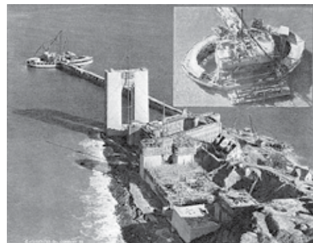
South Anchorage & Tower. Courtesy of Associated Oil Company.
