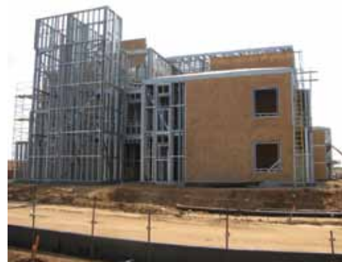
CFS framed structure. Courtesy of Don Allen of DSi Engineering.
