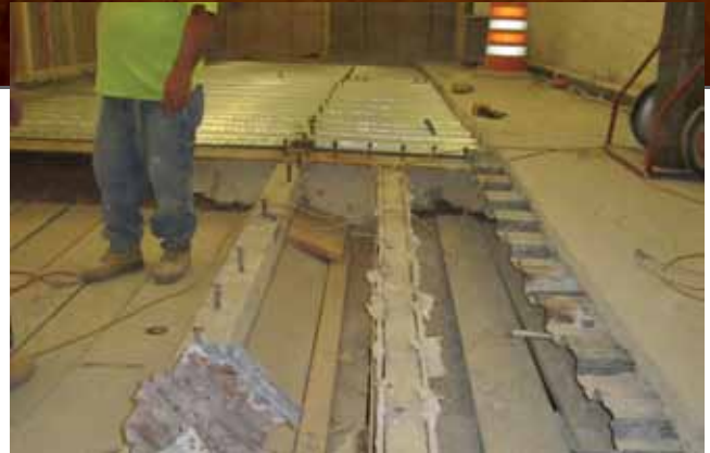
Ramp Renovation in Progress.
