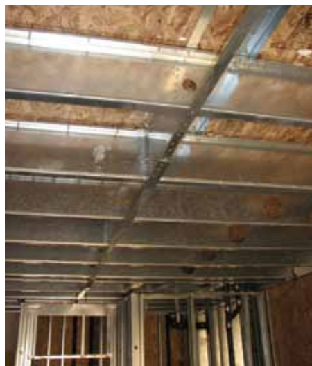
Figure 3: Blocked wood sheathed CFS framed diaphragm. Courtesy of Don Allen of DSi Engineering.
